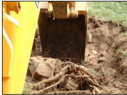
Excavation. Source: http://www.sxc.hu/photo/279748
