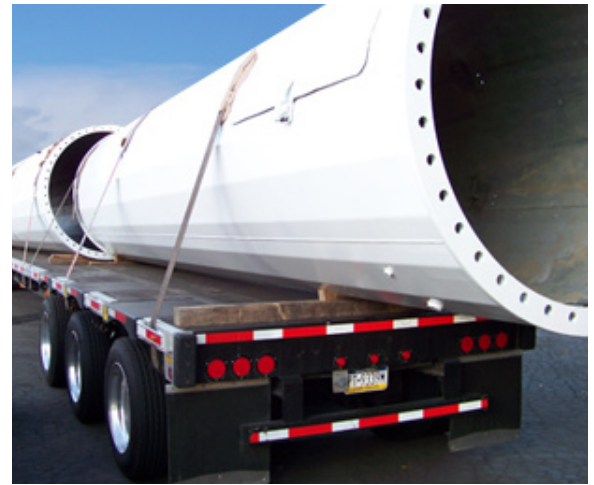
Wind turbine components en route to the Great Escape restaurant, which purchased used parts to save costs. The wind turbine tower reaches roughly 11 stories into the sky.
