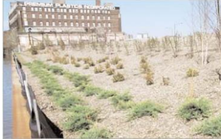
Example of phytoremediation that reduces soil erosion to the river. Source: City of Chicago Brownfields Initiative.
